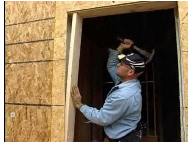
DOOR AND WINDOW FRAMING
